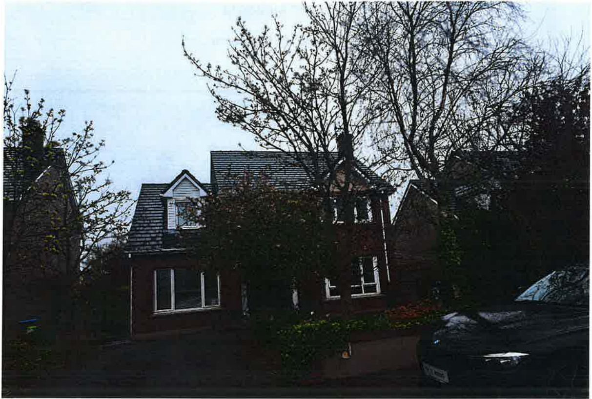
House next door with similar works carried out.
