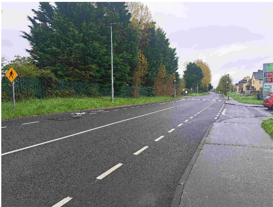
Figure 3.1: R469 Quin Road Resurfacing Complete
