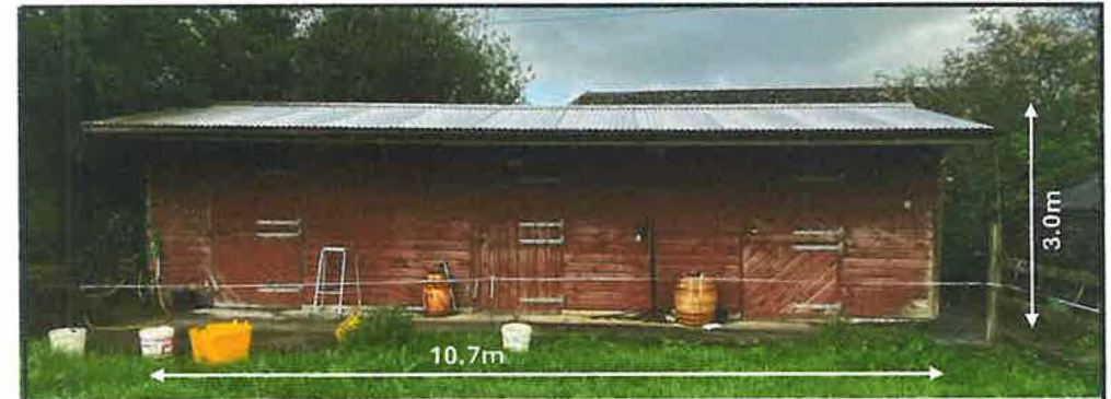
Front View of detached Tool Shed & Stables
