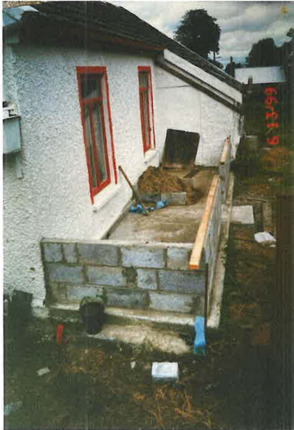
Historic Photograph of Conservatory Annex under construction in 1999
