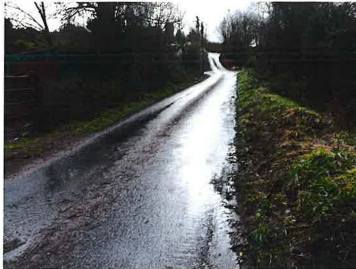
Figure 2: Local Road onto which the existing agricultural access gate is located.
