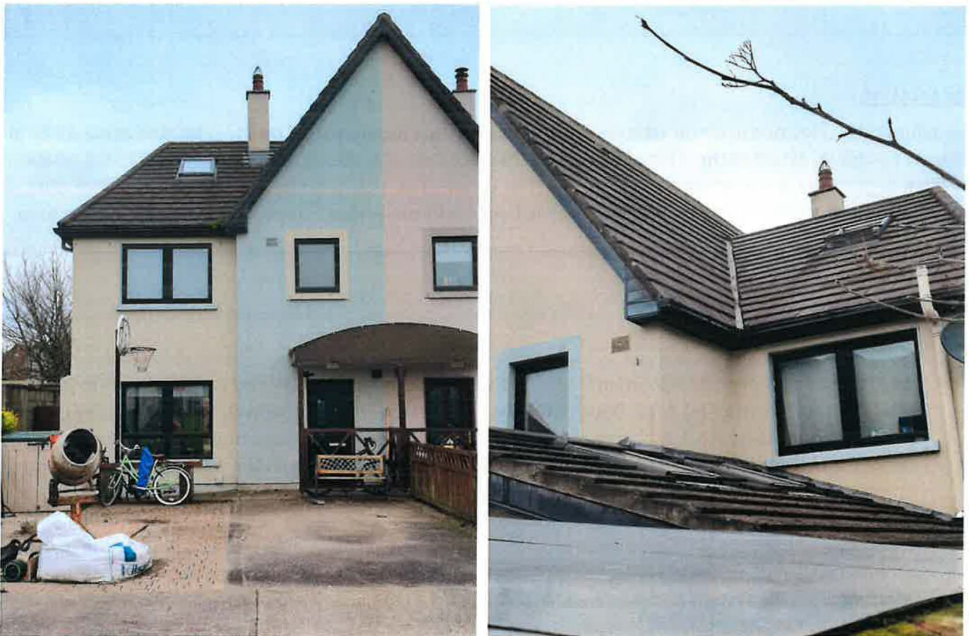
Figure 1: Site as inspected on 08/11/2024
