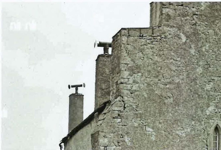
Detail of the North side showing chimney stacks, circa early 20th century, Note the unusual wind/rain cowling solution. Source: Lawrence Collection NLI.
