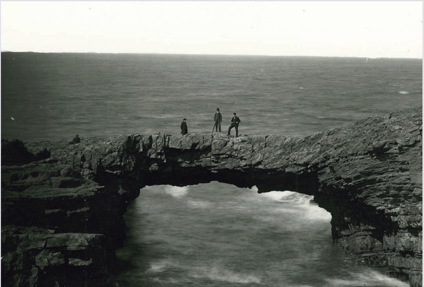
Bridges of Ross
