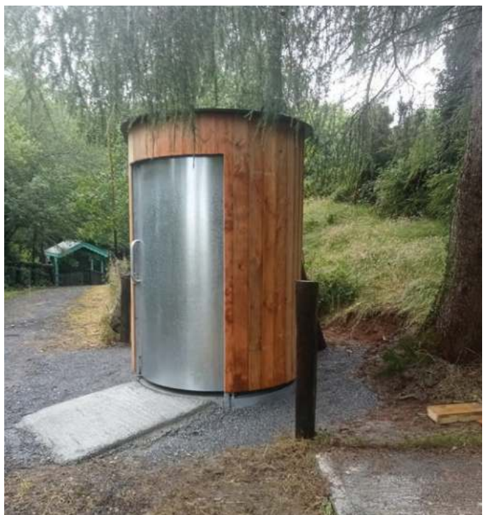
Eco toilet facility at Lissycasey Cascades which received funding of €15,000 under CRF.
