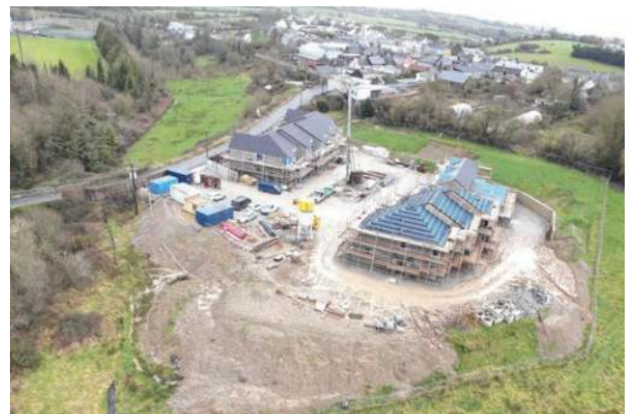
Progress on Scarriff housing development.
