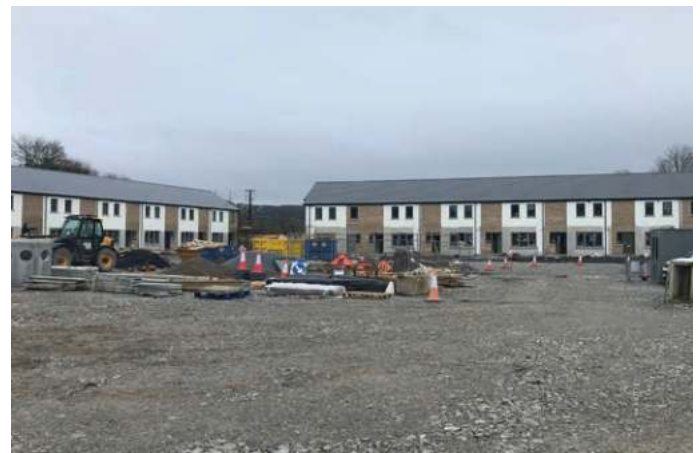
Progress on Sixmilebridge project.
