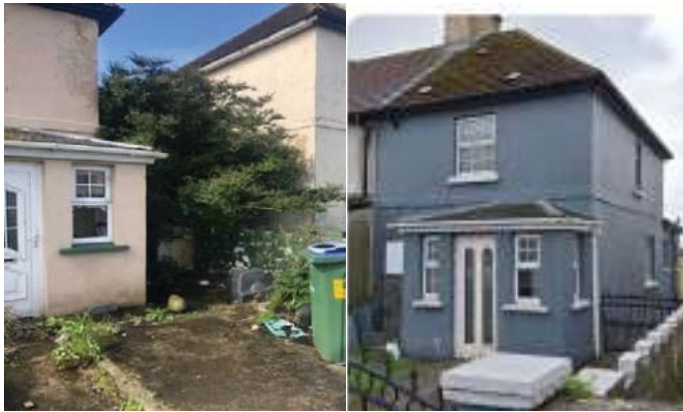
Left: Property in Kilrush (before). Right: Property in Kilrush (after).
