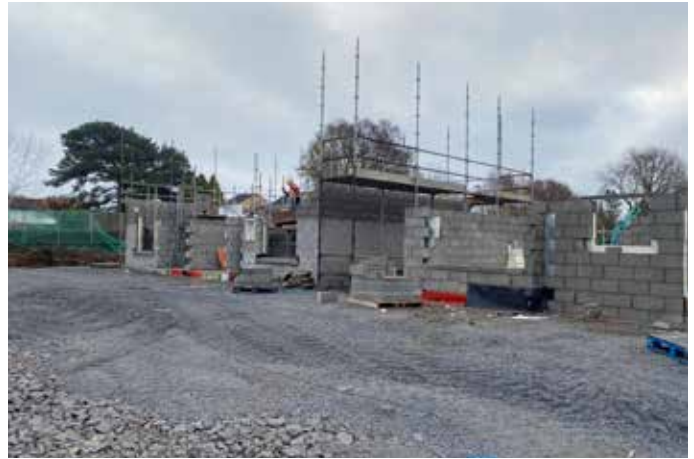
Progress on Gort Road housing development
