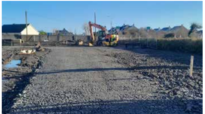
Progress on Doonbeg housing development
