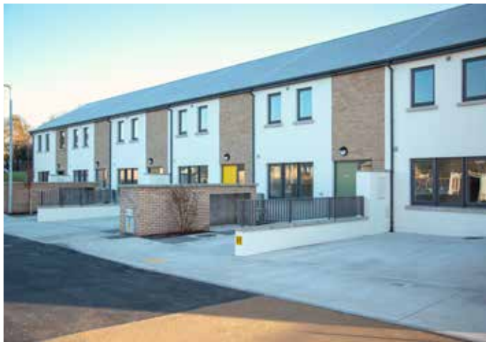
Completed Sixmilebridge housing project
