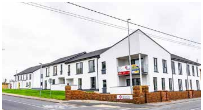
Completed 12 units by Saint Vincent de Paul at Clonroad, Ennis
