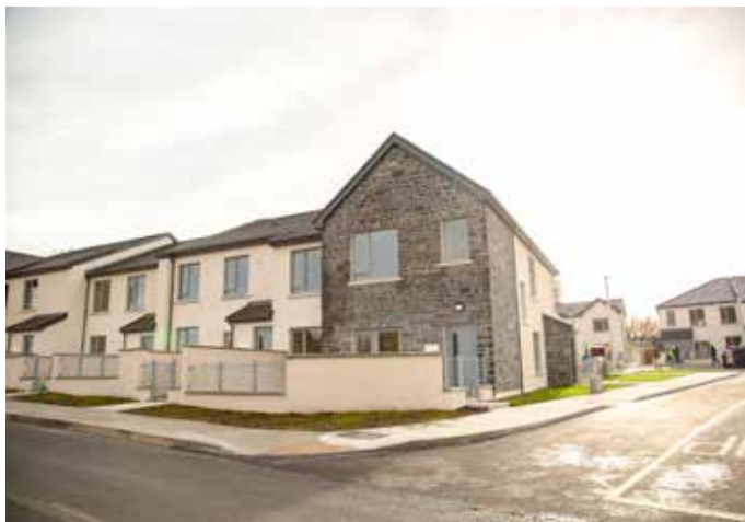
Completed Scarriff housing project
