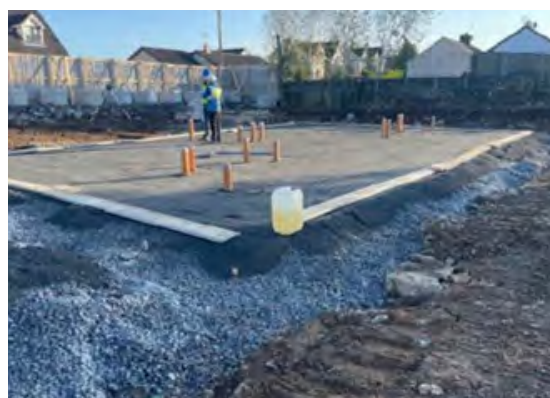
Progress on Gort Road housing development
