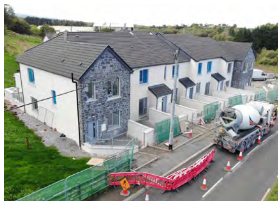
Progress on Scarriff housing development
