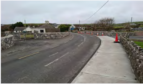
Footpath Works - Roadford ,Doolin
