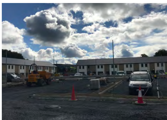
Progress on Sixmilebridge project
