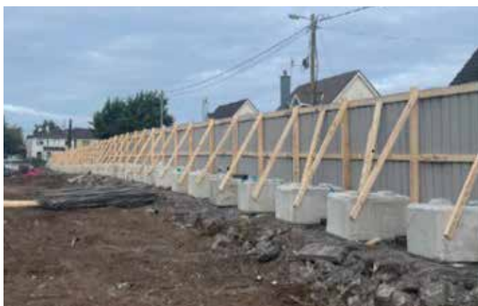
Progress on Gort Road housing development
