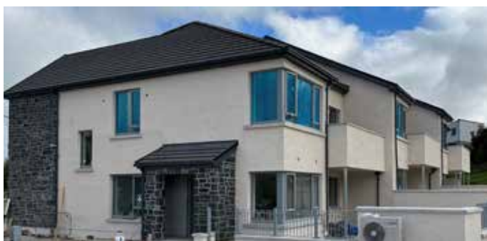
Progress on Scarriff housing development
