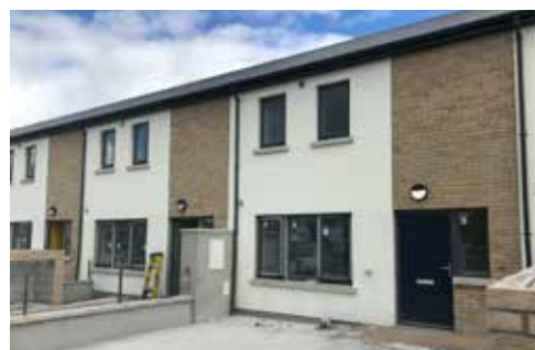
Progress on Sixmilebridge project
