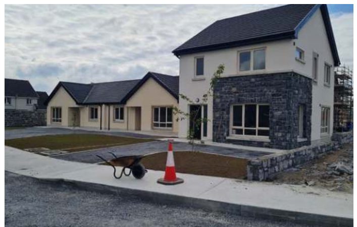
2-bed bungalows at Crusheen provided by Cluid Housing Association
