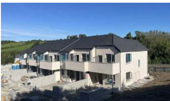
Progress on Scarriff housing development
