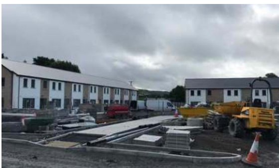
Progress on Sixmilebridge project
