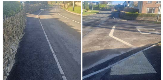
Footpath Refurbishment at no. 3 to 7 at Fairyfield, Parteen. These works included drop kerbs and tactile paving at the entrance into the estate.
