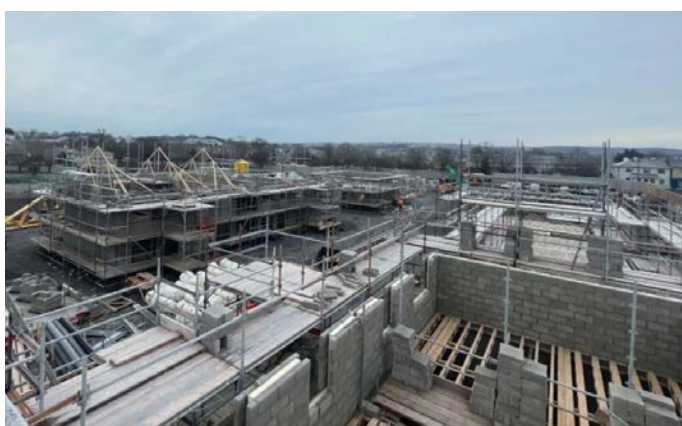
Progress on Gort Road housing development
