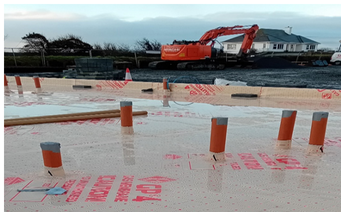
Progress on Doonbeg housing development
