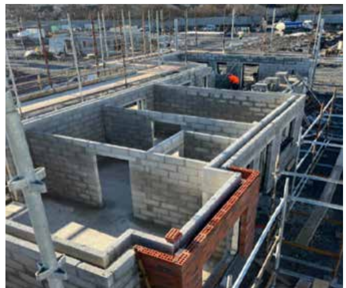
Progress on Gort Road housing development
