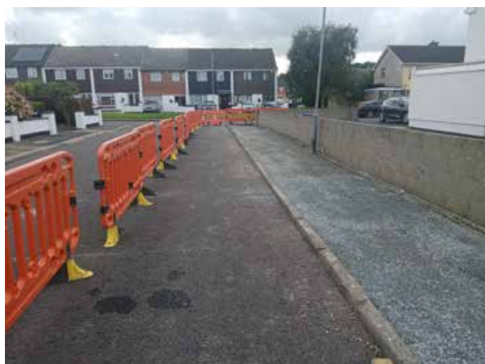
Footpath refurbishment programme at Shannon Walk, Shannon Banks and new footpath Shannon Banks, Corbally.
