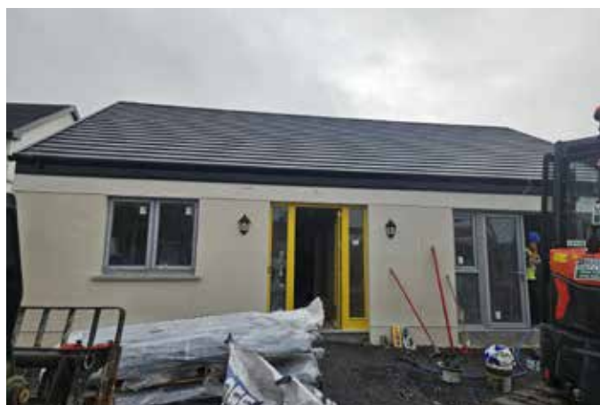
Progress on Shallee/Cloughleigh housing development
