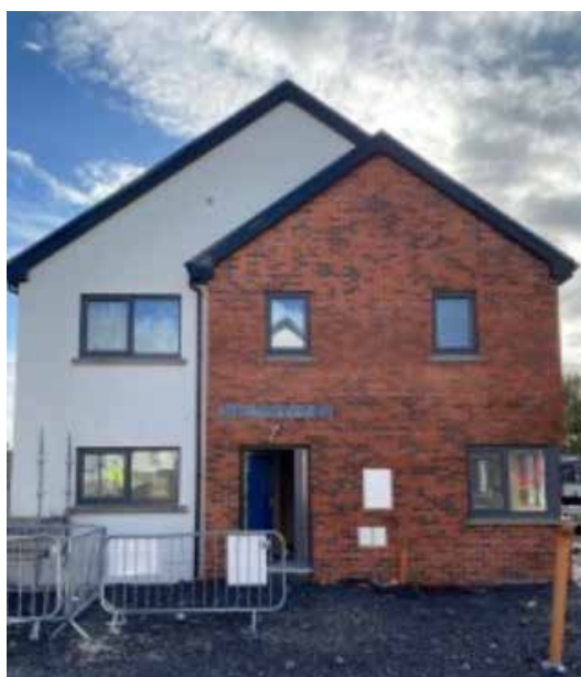
Progress on Gort Road, Ennis housing development
