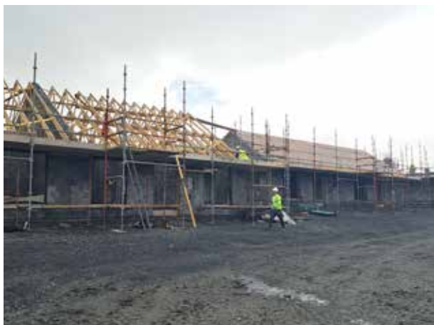
Progress on Back Road, Kilrush housing development
