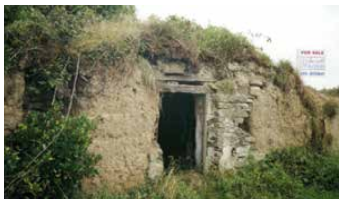
Partial mud house at Johnny Macks Cross in Tullaroe, Querrin prior to the road improvement works.
