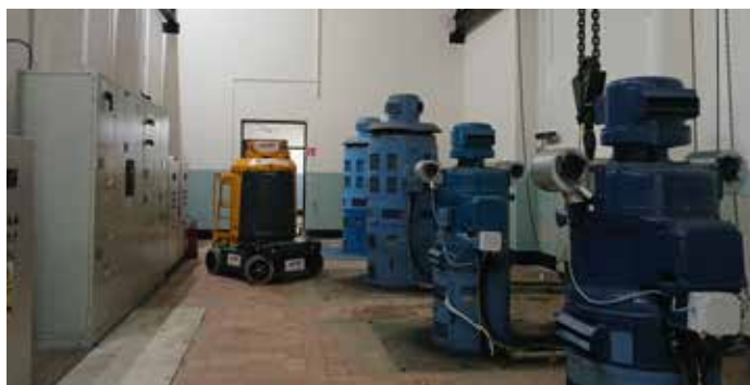
New internal and external lights to Storm Pump House Six, Shannon.
