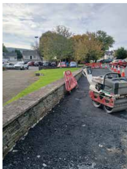
Footpath works at Churchview Sixmilebridge.
