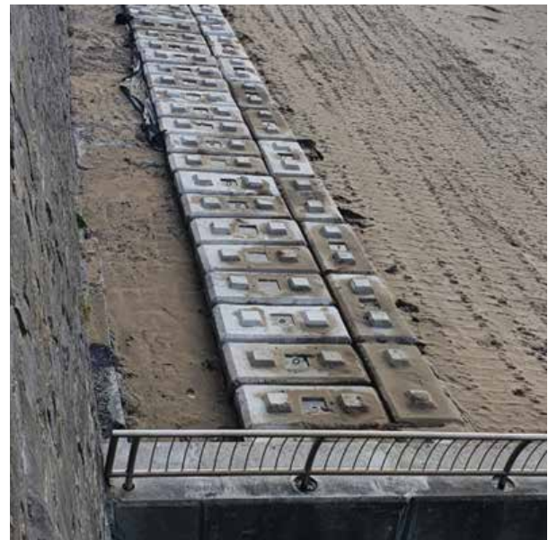
Some preparatory works carried out by Clare County Council. Concrete blocks purchased and placed in position by contractor.
