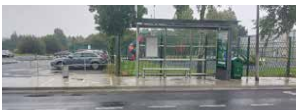
Accessible bus shelter with designated clearance area, access ramp and kerb height for bus access.
